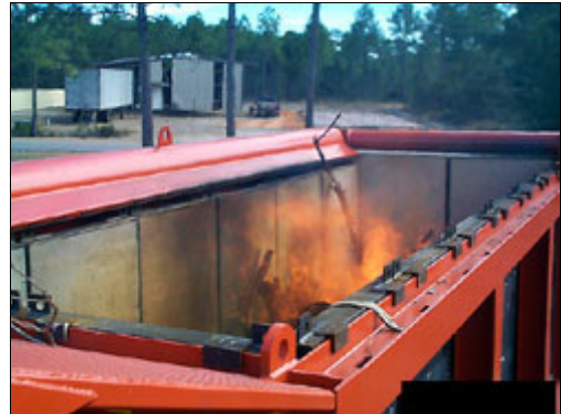
S-116 - Full Operation at Alabama Landfill
