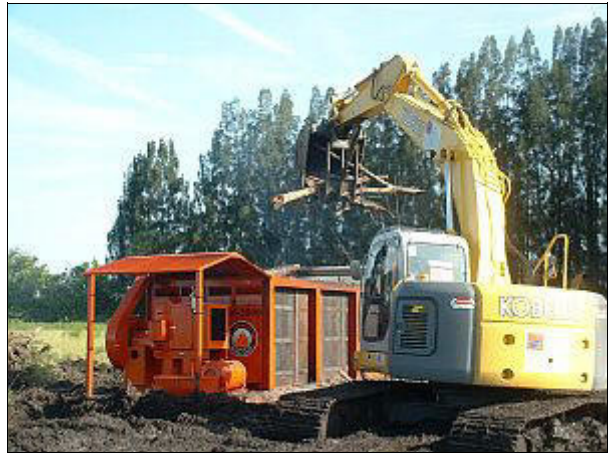
S-217 at Land Clearing Site in Florida
